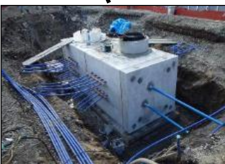
Heat pump using underground heat
