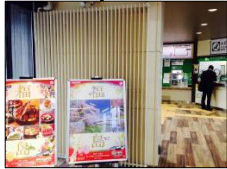
Radiation-type heater using hot spring heat
