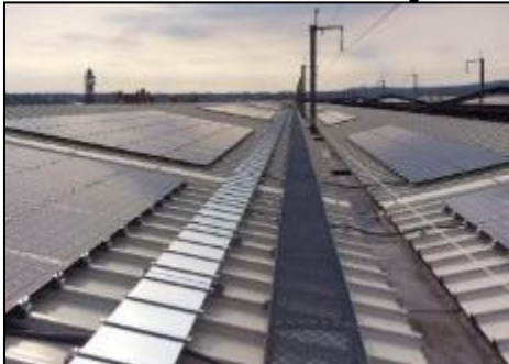
Solar power generation on the rooftop
