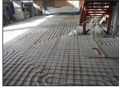
Floor heater using hot spring heat
