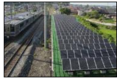
Solar power generation
