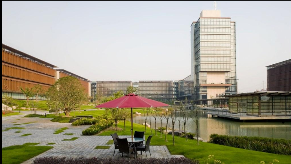
Agricultural Bank of China Data Center, Shanghai, China
