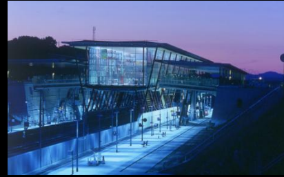
Valence TGV station, France
