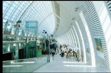
Avignon TGV station, France
