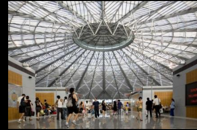
Shanghai South station, China
