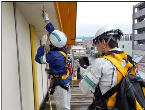
Inspection using fiber scope
