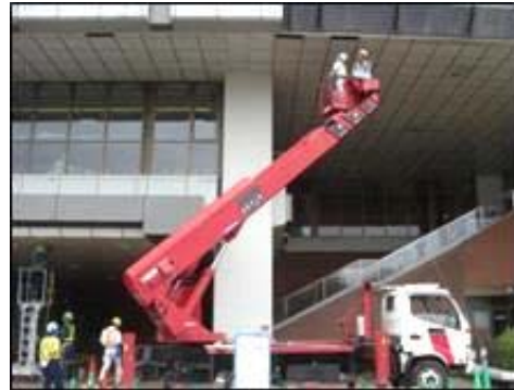
Inspection using vehicle for high lift work
