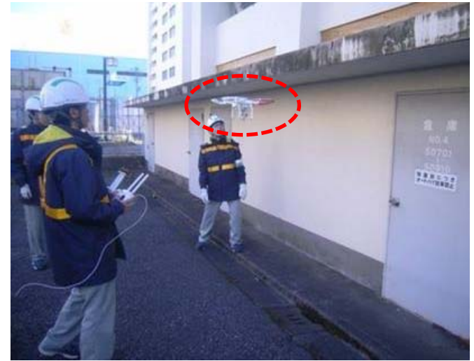
Test of drone for inspection of wall
